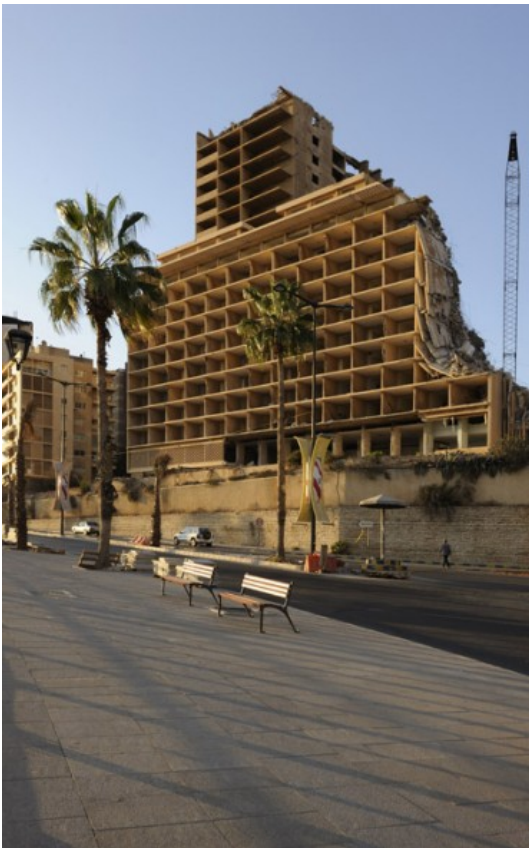
BEIRUT, CARLTON HOTEL, RECENTLY IN DEMOLITION
