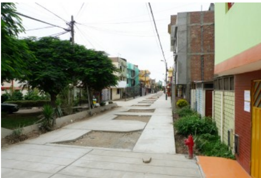
CONCRETE PAVEMENT (PHOTO FROM SEMINARWEEK FS12, NICOLAS HUNKELER)
