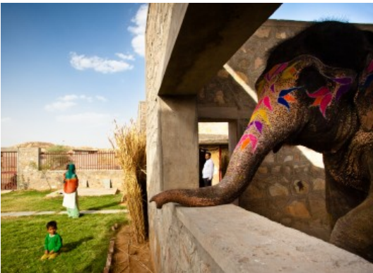
HATHIGAON: HOUSING FOR ELEPHANTS AND THEIR KEEPERS; JAIPUR, RAJASTHAN, INDIA, 2010 PHOTO: CARLOS CHEN
