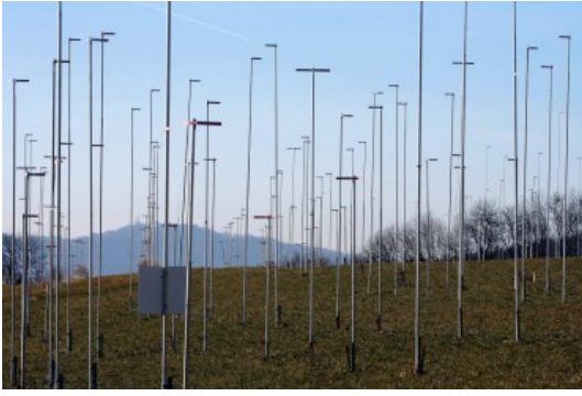
BAUGESPANN TO OUTLINE THE BUILDING VOLUME PRIOR TO THE START OF CONSTRUCTION PHOTO: ALESSANDRO DELLA BELLA, ZUMIKON, 2008
