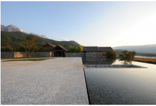
WATER HOUSE, LIJIANG, CHINA
