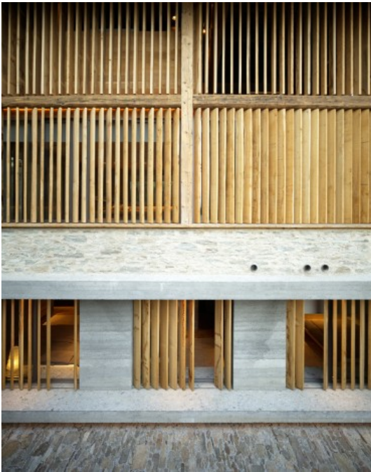
RENOVATION OF A STABLE IN SOGLIO, 2009. RUINELLI ASSOCIATI ARCHITETTI
