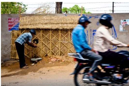
THATCHED HUT USING PASSIVE COOLING TECHNIQUES TO KEEP DRINKING WATER COOL FOR PUBLIC SUPPLY PHOTO: CARLOS CHEN
